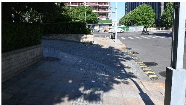
Figure 7: Excessively steep road gradient Self-photography
