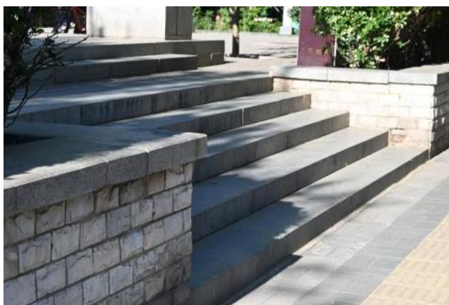
Figure 13: Lack of accessible ramps Self-photography
