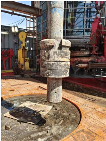
Figure 6: Diagram of the integrated tool for wellhead flushing and fishing with a fishing sleeve out of the well
