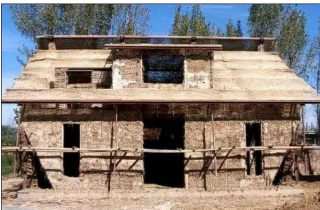
Figure 2: Application of Straw Bricks in Building Structures
