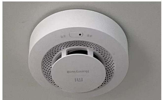
Figure 9: Smoke and fire sensing alarm
