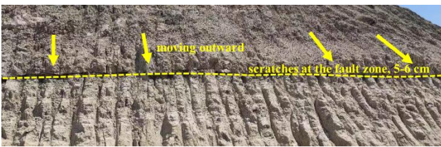
Figure 14: Displacement at the Front Edge of the Composite Slope
