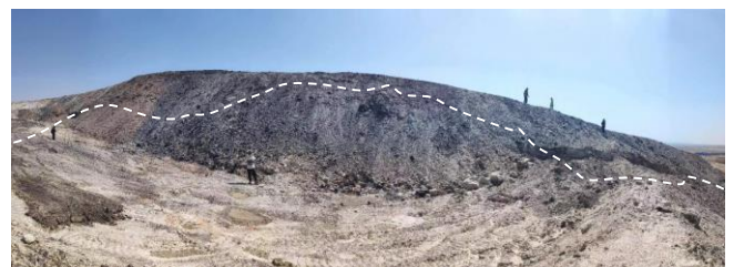
Figure 12: Panoramic View of the Back Edge Fracture of the Composite Slope
