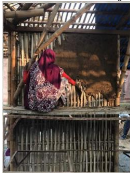
Figure: Daub walls construction
