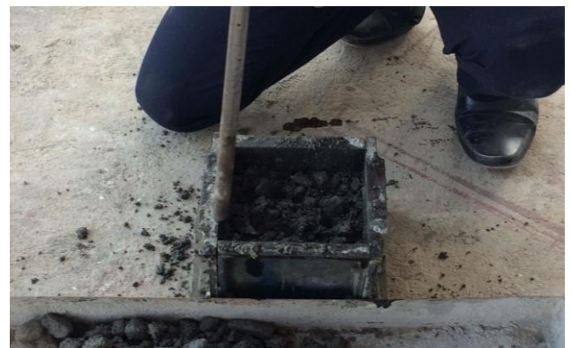
Figure 15: Compacting the concrete in the cube mould (For 150 mm cube at least 25 tamps per layer)
