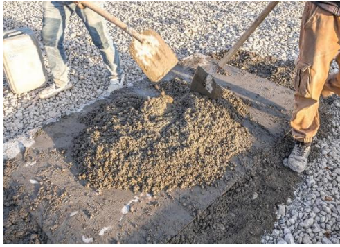
Figure 12: Mixing of concrete
