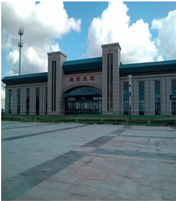
(a) Fuyu North Station
