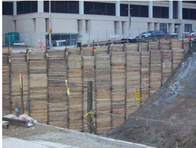
Photo 2: Tieback through pile penetration
