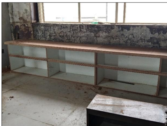
Figure 3: Condition of the Window Wall on Level 2
