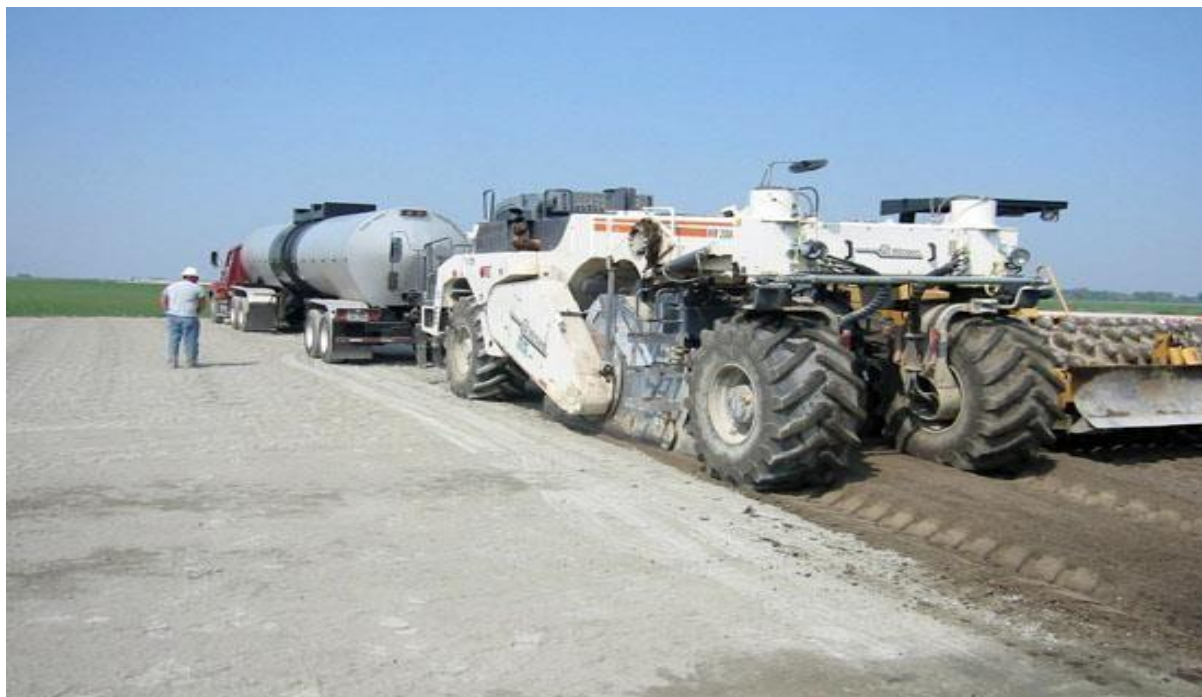
Figure 2.3: Rejuvenating existing pavement structure by stabilizing for FDR
