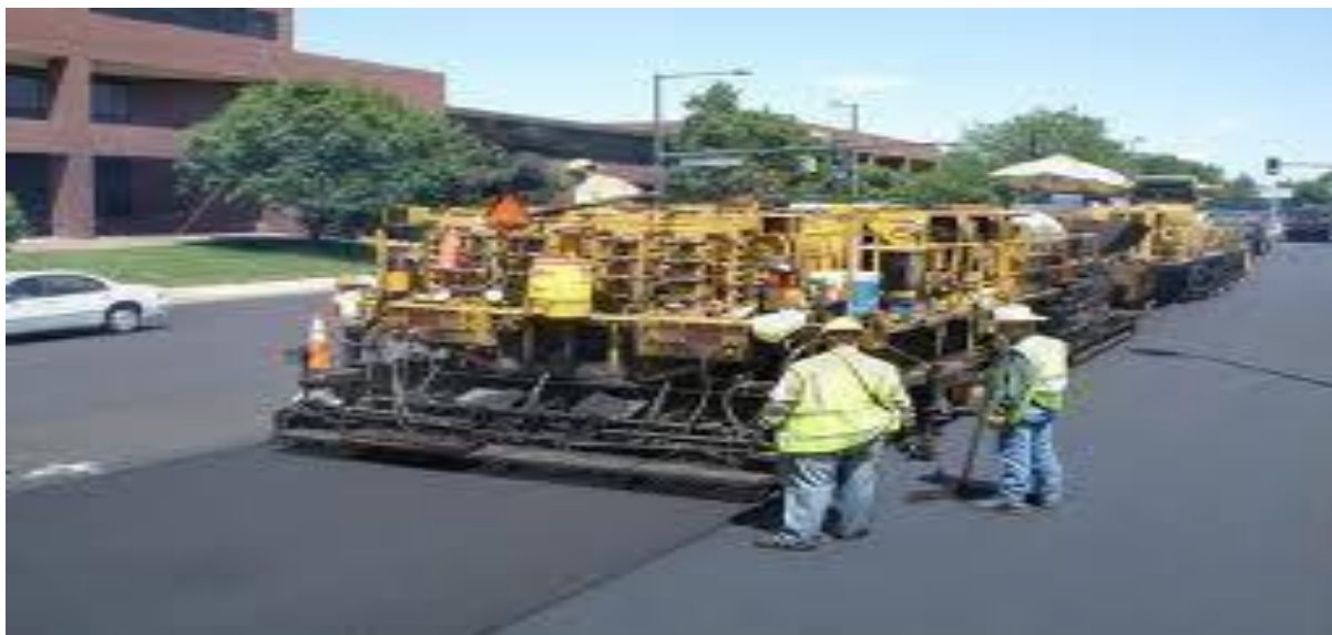
Figure 2.1: Hot in place recycling
