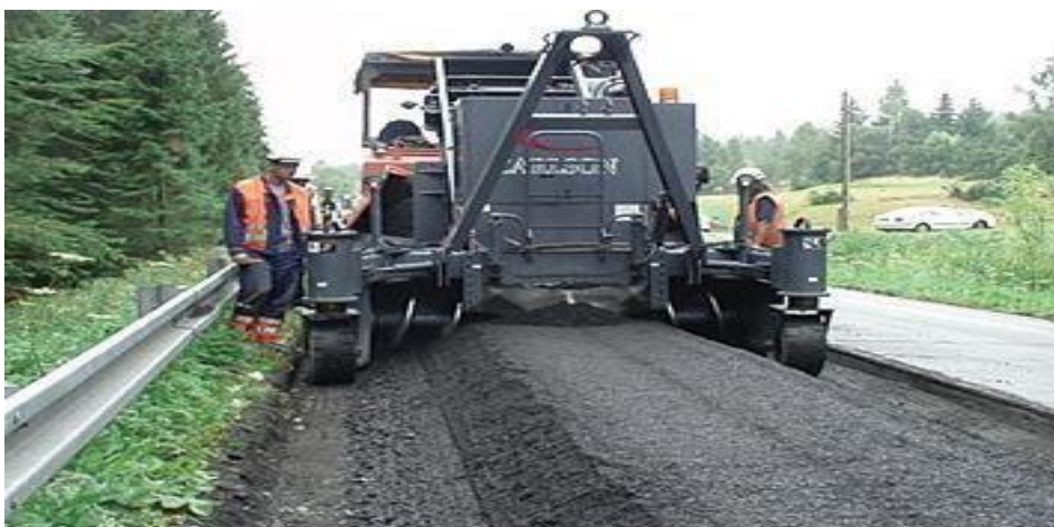
Figure 2.2: After being processed, the material is deposited onto the roadway in a windrow
