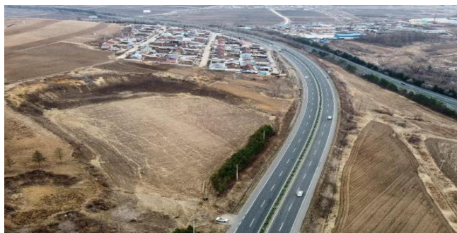
Figure 1: Sampling point topography and expansion contraction cracking situation
