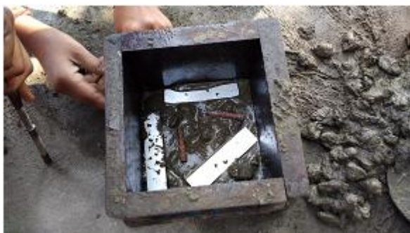
Figure 2: Concrete cube casting
